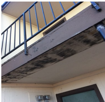
8 20 Unit 277 Patio/Porch/Balcony - Ceiling
