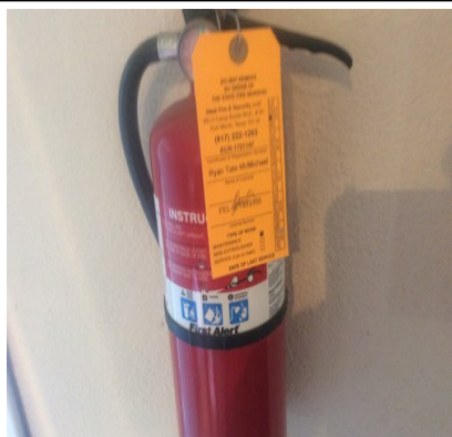
1 1 Fire Protection - Extinguisher
