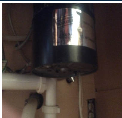
2 13 Unit 156 Kitchen - Dishwasher/Disposal
