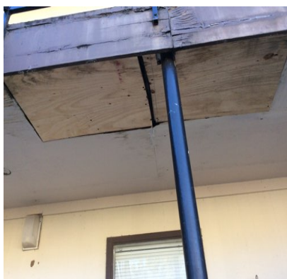
11 8 Unit 91 Patio/Porch/Balcony - Ceiling
