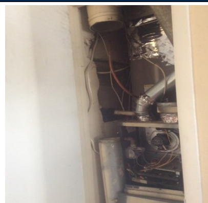
4 9 Unit 106 Local Systems - HVAC System
